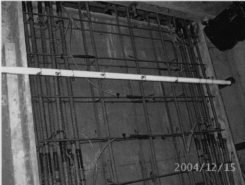
Figure 3. 4 Wall reinforcement details
