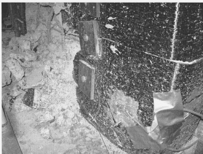
Figure 4- 78 Wall RW9 failure.
