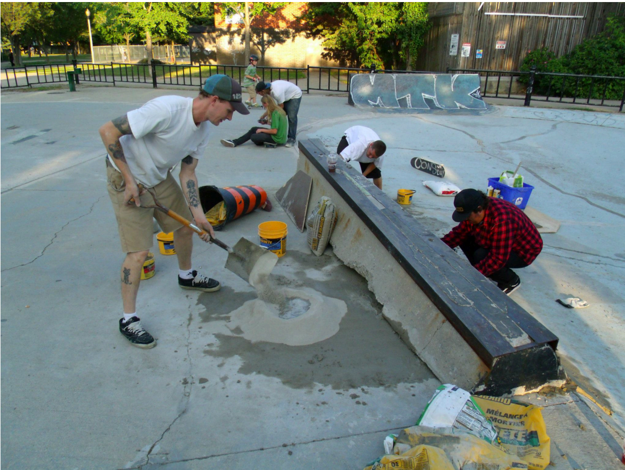
Figure 14. Skateboarders adding a concrete transition to a Jersey barrier. 2012 Photo by Simon Orpana.
