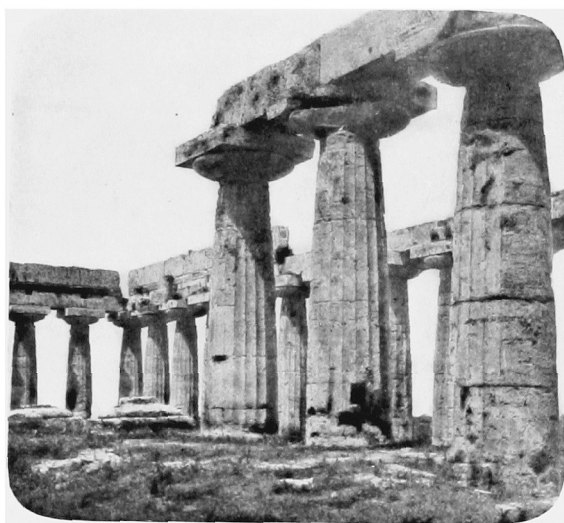
Fig. 77. The Entasis at Pæstum. The so-called Basilica, a Sixth-century Temple.
