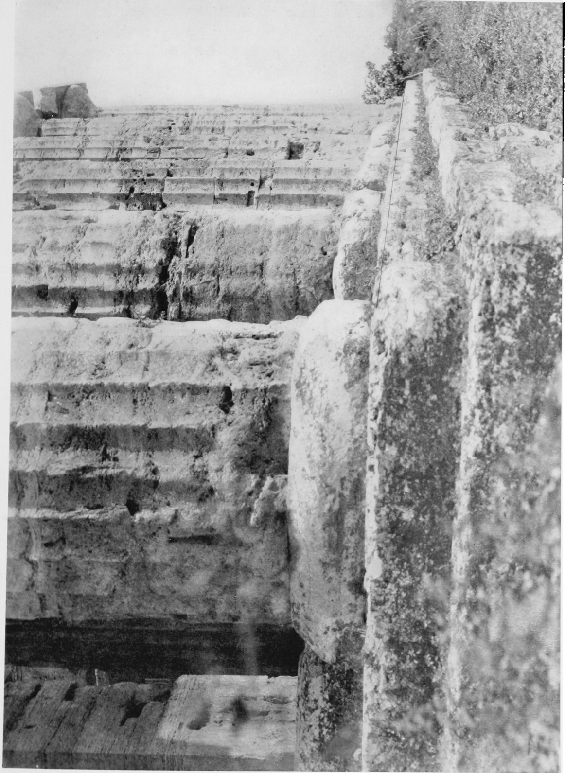
Fig. 54. Curve in Elevation, Stylobate of the Temple of Poseidon at Paestum, East Front. Brooklyn Institute Museum Series of 1895. A straight line has been drawn on the upper step in order to show the curvature, which has a deflection of 2 cm., or \frac{3}{4} inch, in 80 feet.
