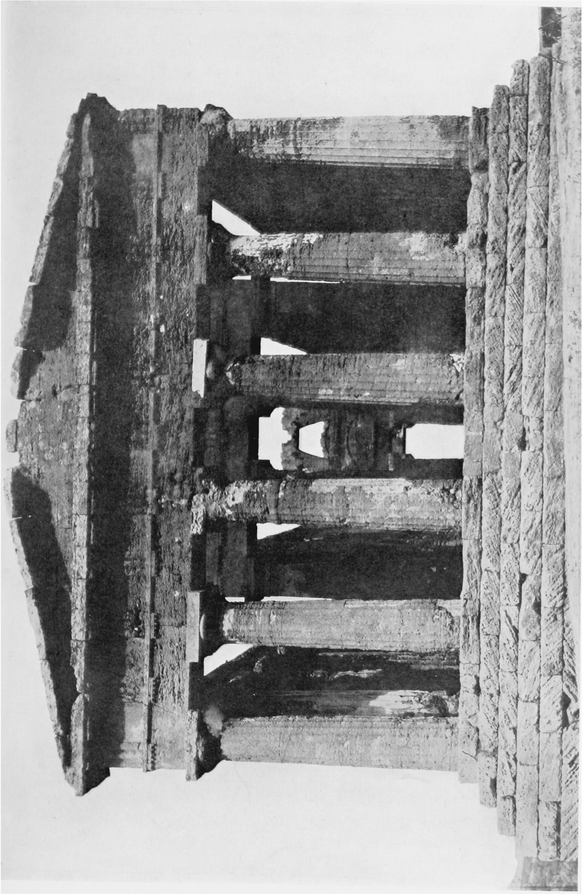
Fig. 41. Temple of Concord at Girgenti. West Front, in Parallel Perspective. Showing the absence of curvature in the stylobate and in the entablature. Brooklyn Institute Museum photograph, series of 1895.
