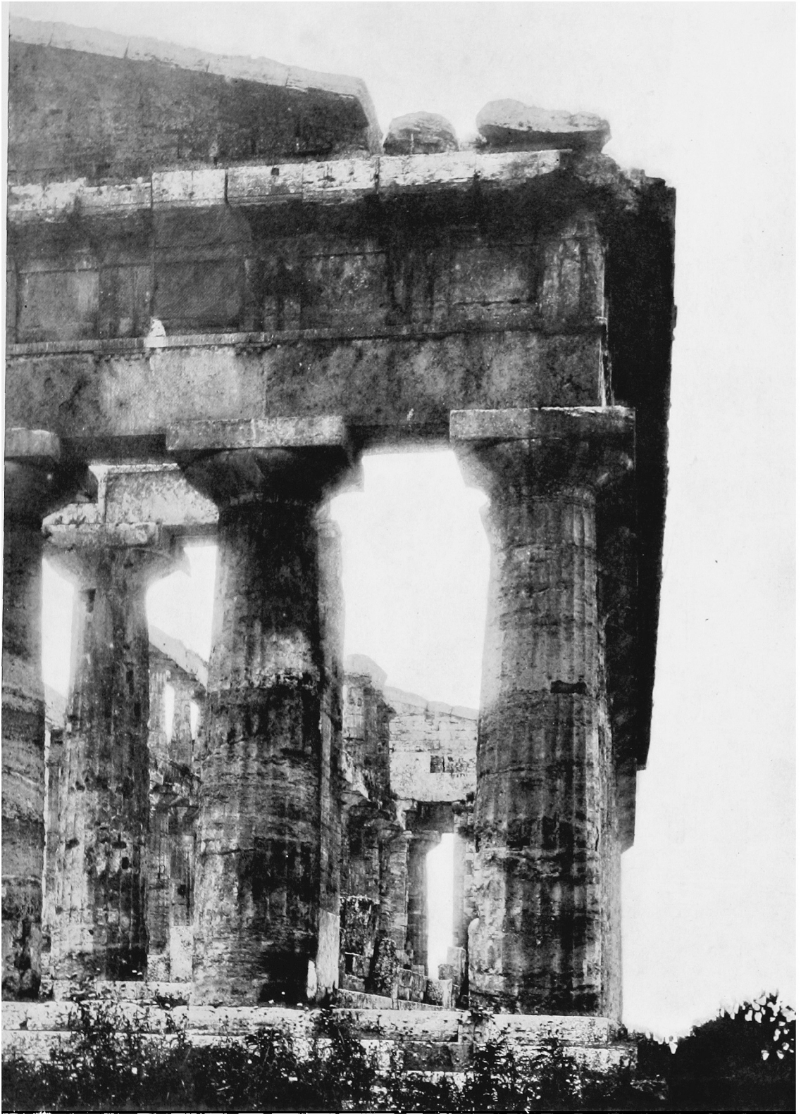
Fig. 26. North Flank of the so-called Temple of Poseidon at Paestum. Fifth Century B.C. Curves in plan in the capitals and cornice. Brooklyn Institute Museum photograph, series of 1895. The cornice curve is best sighted by holding the page upside down.
