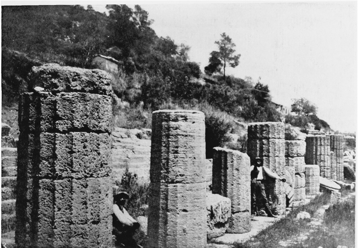
Figs. 93, 94. Temple of Hera at Olympia. Asymmetric Columns of the North Flank.
