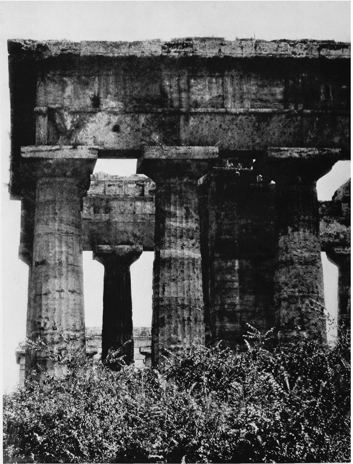
Fig. 1. Curves in Plan, Concave to Exterior, in Capitals and Entablature.
