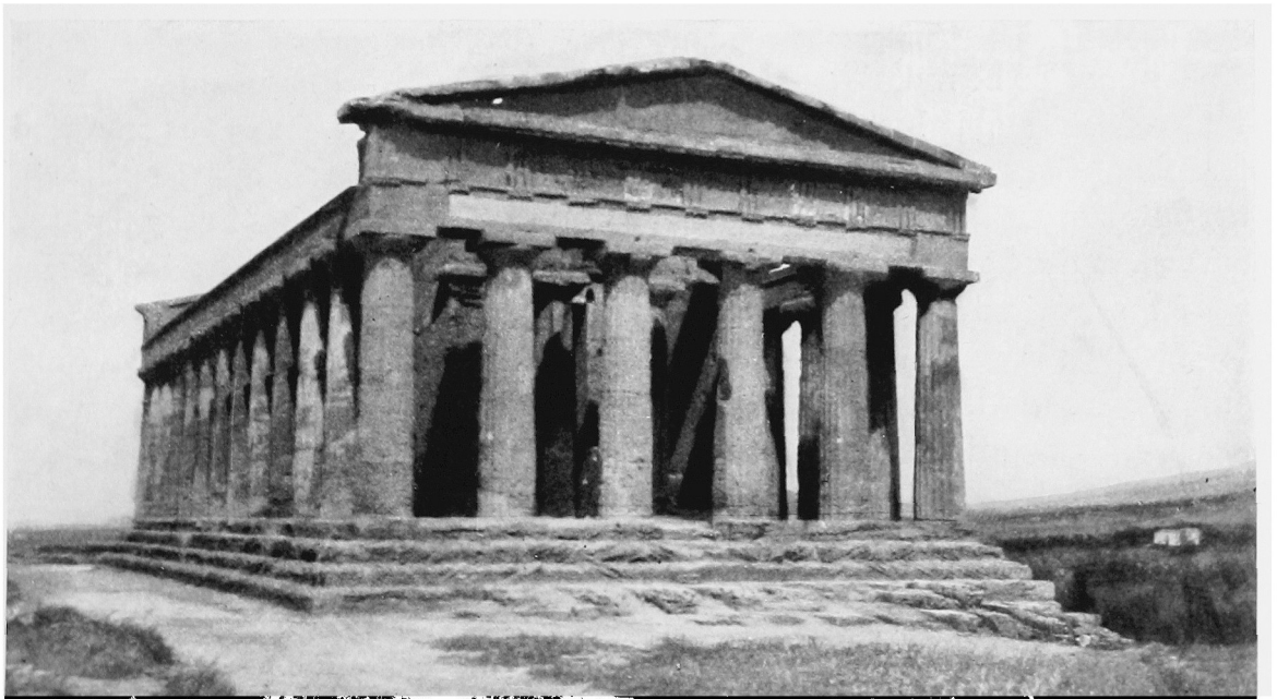
Fig. 39. Temple of Concord at Girgenti, showing Curves in Elevation on the South Flank Stylobate.
