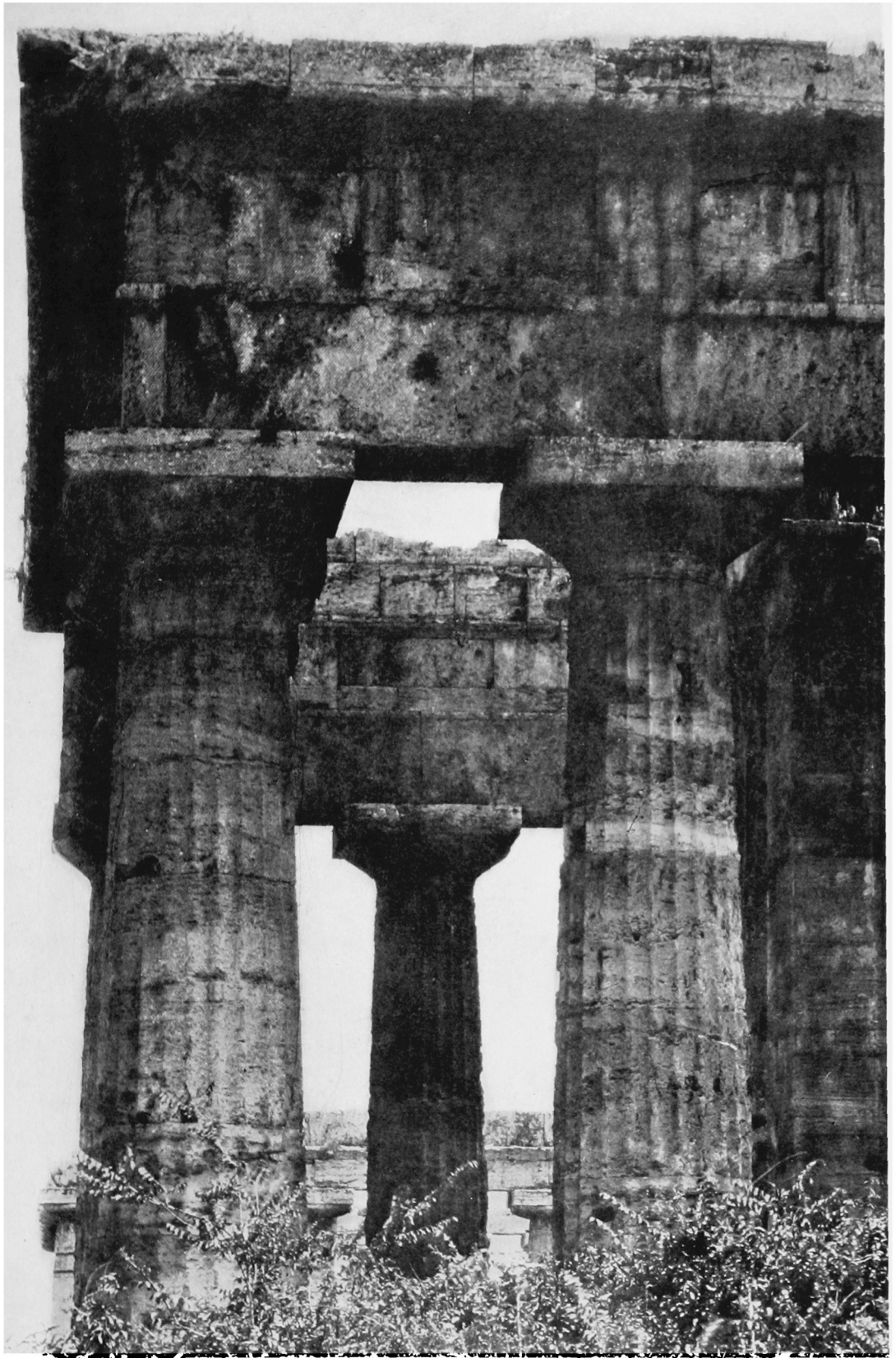
Fig. 33. Concave Curvature. East Front of the so-called Temple of Poseidon at Paestum. The curves occur in the alignment of the capitals and in the entablature. From a Brooklyn Institute Museum photograph, series of 1895.
