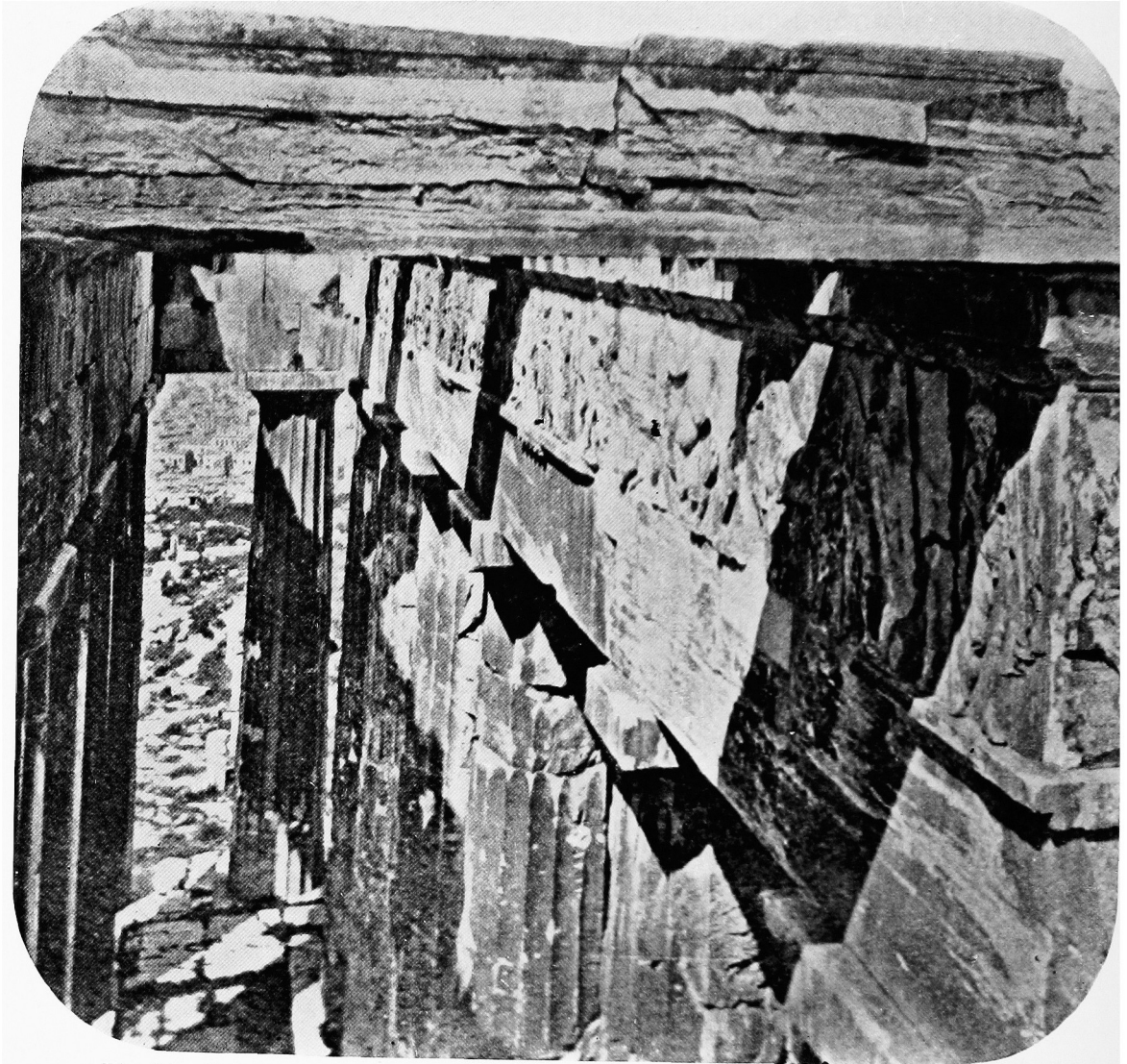
Fig. 14. Curves of the Parthenon, Entablature of the Inner Portico, West Front. Commercial photograph.
