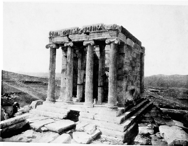
Fig. 74. Temple of Nike Apteros, Athenian Acropolis. Fifth Century B.C. This temple had no horizontal curvature, according to Penrose. It was rebuilt in 1835-6, with the original masonry, which had been used for a fortification by the Turks.
