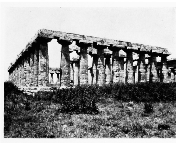
Fig. 83. The Doric Columnar Diminution. The so-called Basilica at Paestum.
