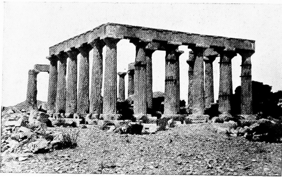
Fig. 68. Temple Ruin, Ægina. Fifth Century B.C. This temple has no horizontal curvature.
