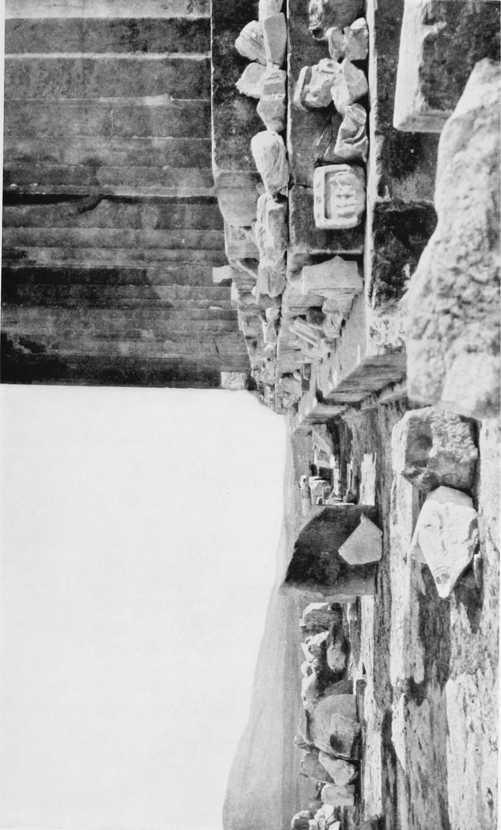
Fig. 50. Curves in Elevation of the Stylobate, East Front of the Parthenon. From a Stillman photograph belonging to the Architectural School of Columbia University.
