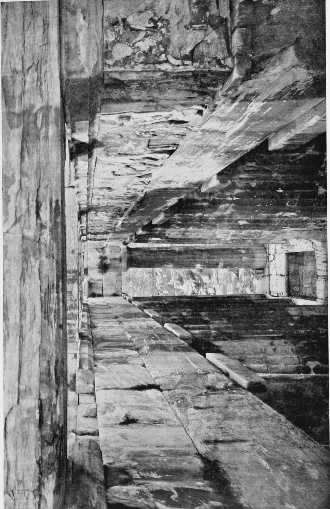
Fig. 51. Curves in Elevation of the Parthenon Frieze, Western Portico; Sighting on the Entablature. From a Stillman photograph belonging to the Architectural School of Columbia University.
