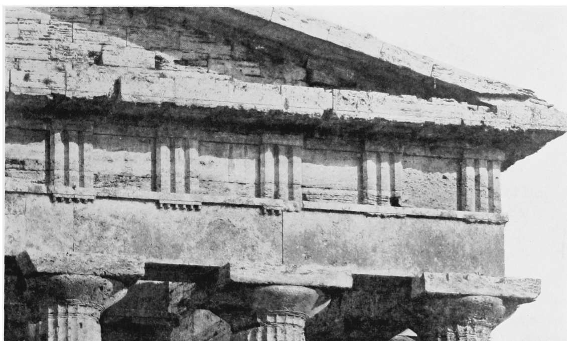
Fig. 12. Entablature and Pediment of the so-called Temple of Poseidon at Paestum. To illustrate the decentering of the angle triglyph, as related to the angle column.
