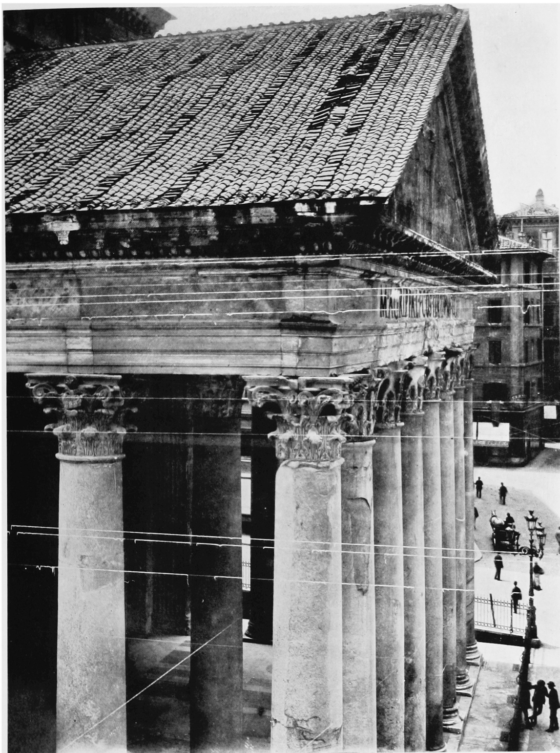
Fig. 76. Curve in Elevation, Front Cornice of the Pantheon.
