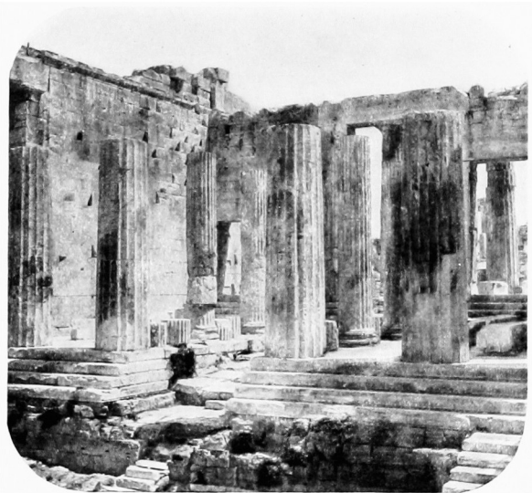
Fig. 67. The Propylæa, Athenian Acropolis. There are horizontal curves in the entablature, but not in the platform, as observed by Penrose.
