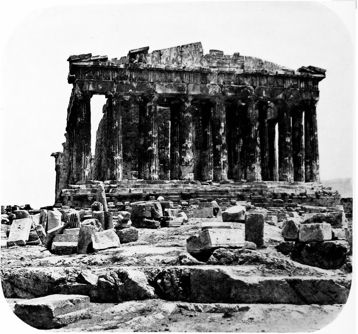
Fig. 3. West Front of the Parthenon.
