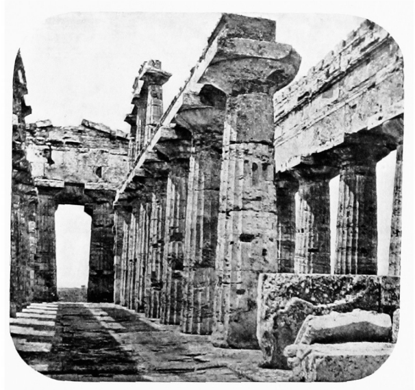
Fig. 82. The Doric Columnar Diminution. Interior of the Temple of Poseidon at Paestum.
