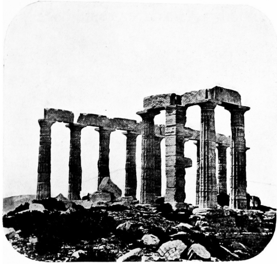
Fig. 63. Temple Ruin at Sunium, Fifth Century B.C. The horizontal curvature has been observed by Penrose.
