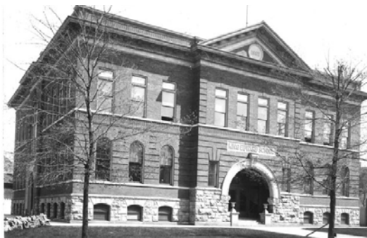
Figure 5.2: Old King Edward School in the Early 1900's in Hamilton (Courtesy of the Educational Archives and Heritage Centre)
