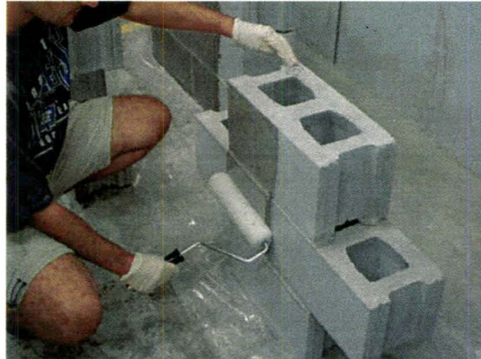
(a) Applying Epoxy to the Specimen
