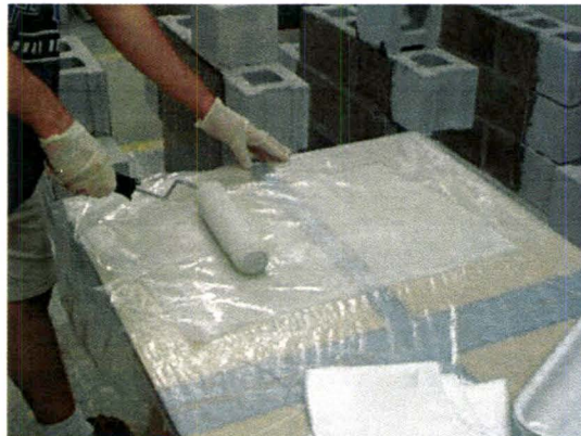
(b) Saturating the Fibreglass Fabric with Epoxy
