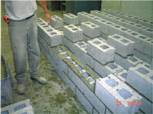
(b) Construction of Specimens in Running Bond
