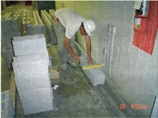
(a) Leveling the First Course
