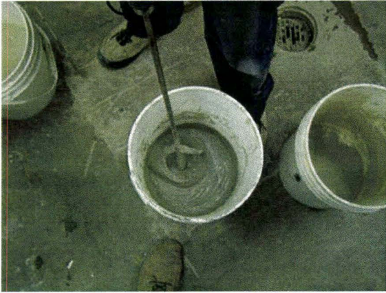
(a) Mixing the Parging
