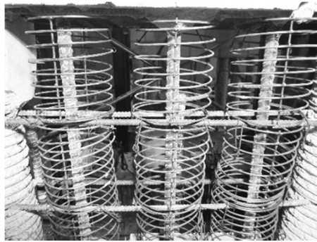
b) Additional Confining Devices and Horizontal Reinforcement
