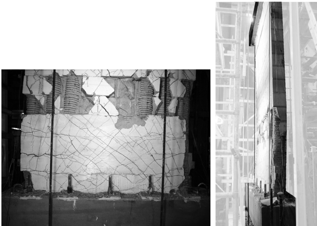
a) Spalling Damage at Wall Ends and at Interface above Repaired Zone
