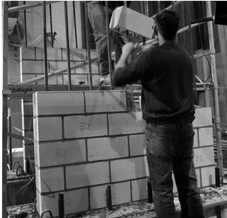
Figure 5.5. Wall Construction: Blocks Being Lowered Over Vertical Reinforcement
