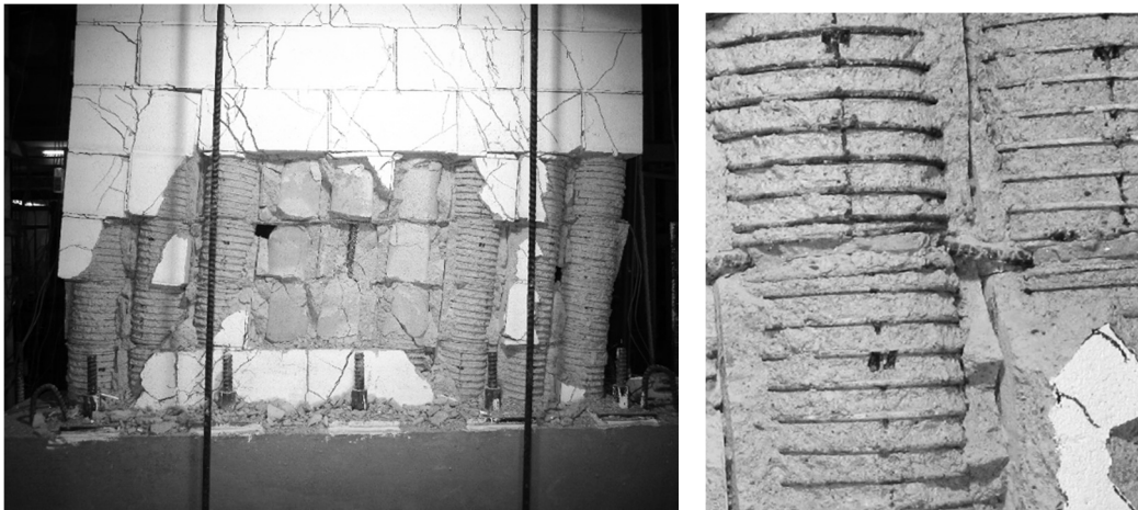
a) Extent of Spalling at Test Completion
