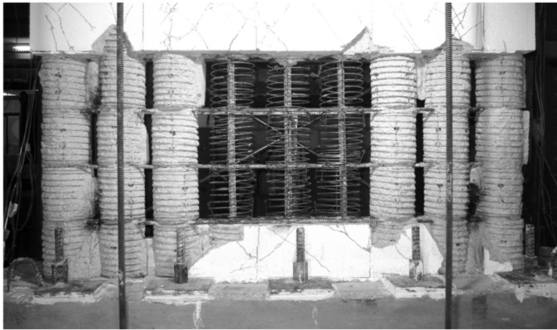
a) Wall Prepared for Retrofit Following Chiseling of Concrete between Confined Grout Columns
