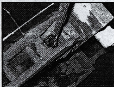
(b) Laying mortar bed joints
