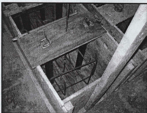
(b) Framework for vertical bars and tubes to accommodate prestressing rod
