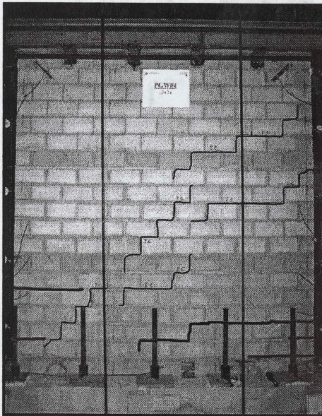
(a) New cracks during 1.00 mm and 1.20 mm displacement cycle
