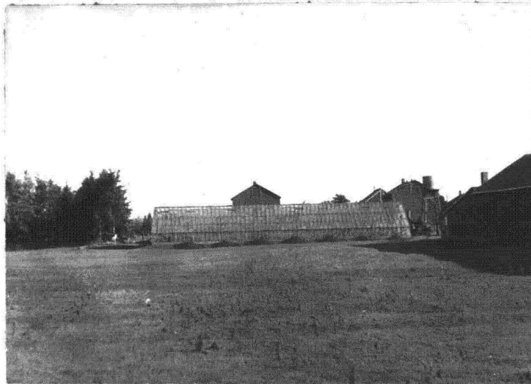
Tobacco Buildings. Note the greenhouse, pack-barn, water tower, kilns and steam engine. Also note used muck beside greenhouse.
