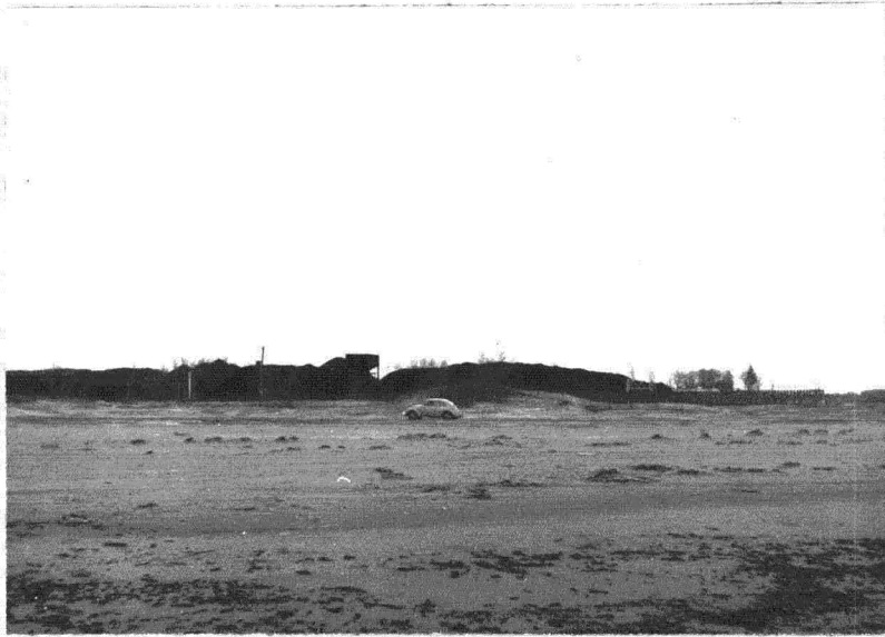
Large Artificial Beach West of Port Burwell, Built by longshore currents and waves after construction of breakwater.
