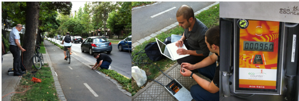
Figure 14. Installation process of Pneumatic Tubes
