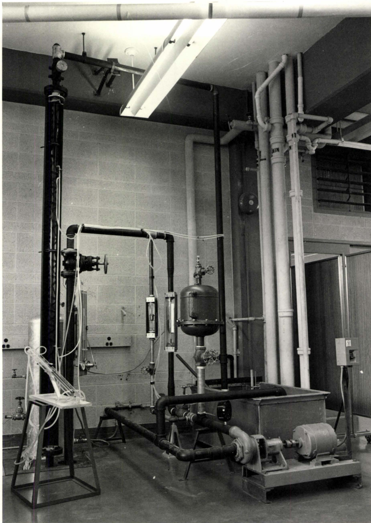
Plate #1 Overall view of apparatus, second floor
