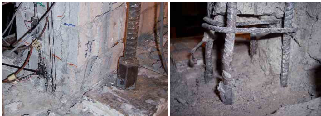
Figure 3.18 – Eventual Fracture of Reinforcement and Failure of Wall 7 in East Toe (Left Photo: \Delta\epsilon = -2.63\% second cycle, Right Photo: \Delta\epsilon = +3.68\% first cycle, grout core removed)
