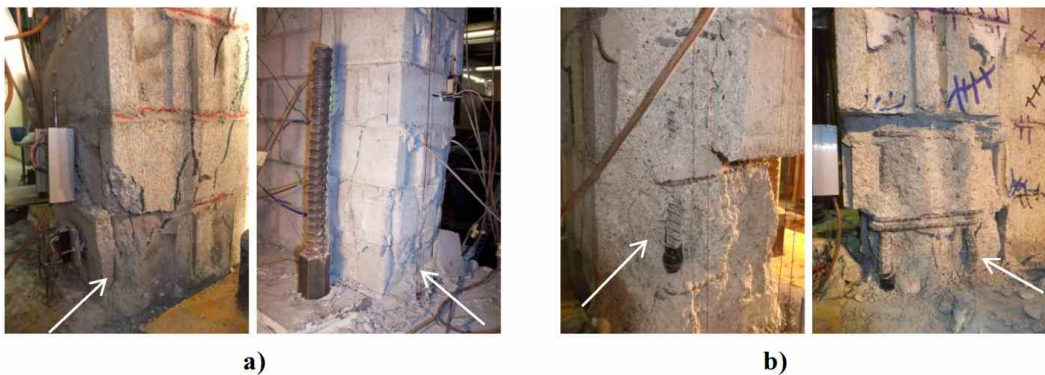
Figure 4.17 – Visual Observation-Based Damage States: a) Spalling of the Face Shell and Vertical Cracking and b) Crushing of the Masonry to Expose Reinforcement
