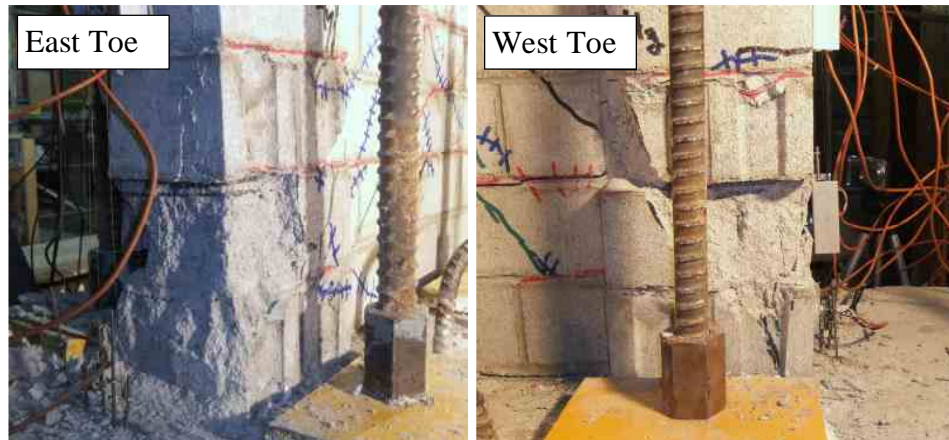
Figure 3.21 – Initiation of Face Shell Spalling in Wall 9 ( \Delta\% = \pm 1.38\% ) with Grouted Core Intact
