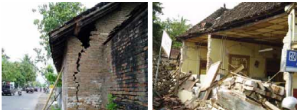
Figure 4.6 Half brick thick masonry building without reinforcements (Boen 2006)
