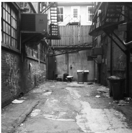
Figure 5.8 Down “Crack Alley” (Author, 2012)
