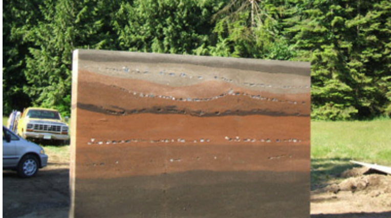
Figure 4: The layers of soil in a rammed earth wall (Schooly, 2008)
