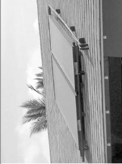
Photo: Roof-mounted, flat panel solar collectors used for heating water (Olsen, 2001)
