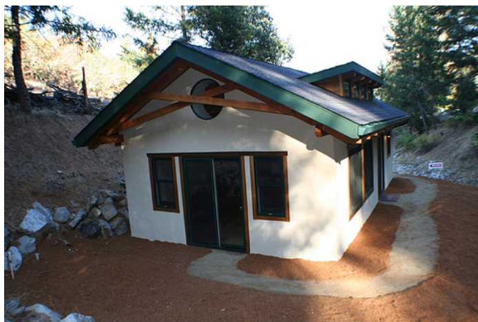
Figure 1: A straw bale cottage about the minimum size recommended for using straw bale, adobe, or rammed earth (StrawBale Innovations, LLC, 2011)
