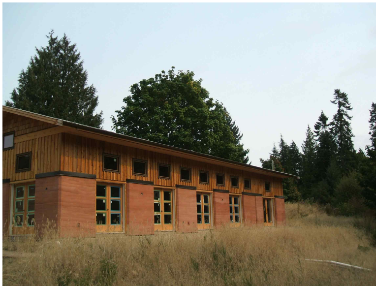
Figure 3: A rammed earth home. Notice how the walls can be sided with wood for a conventional look or left bare to show the rammed earth walls (Schooly, 2008)
