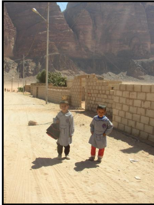
Photograph 3 A typical street in Rum Village in 2002 before the upgrades. Note the above ground power lines and light standards.
