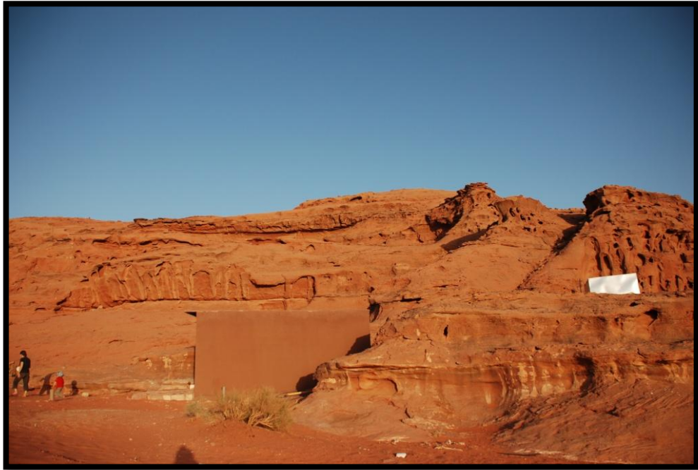
Photograph 7 The finished toilet at Lawrence Camp. This was not a design held in high regard by the owner.
