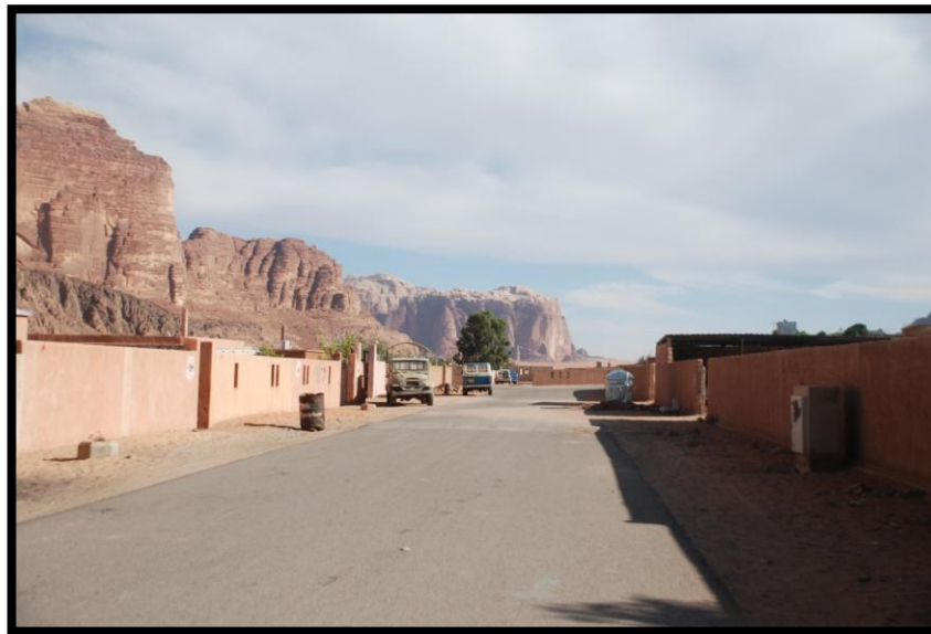
Photograph 4 A street after the upgrades – paved road, walls, light standard (broken on left), garbage bins and underground electrical.
