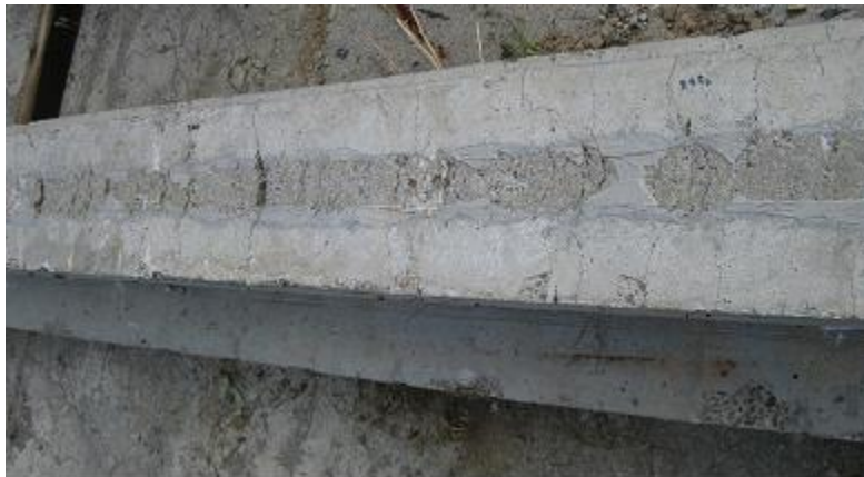
Figure 4.26: Failure plane of east side EB1
