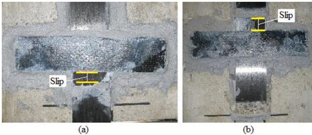
Figure 4.13: Debonding of DS6 (a) Top north face and (b) Bottom south face
