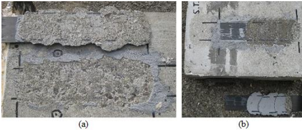
Figure 4.1: Failure plane of (a) Bottom south side of DS1 and (b) Top south side of DS2
