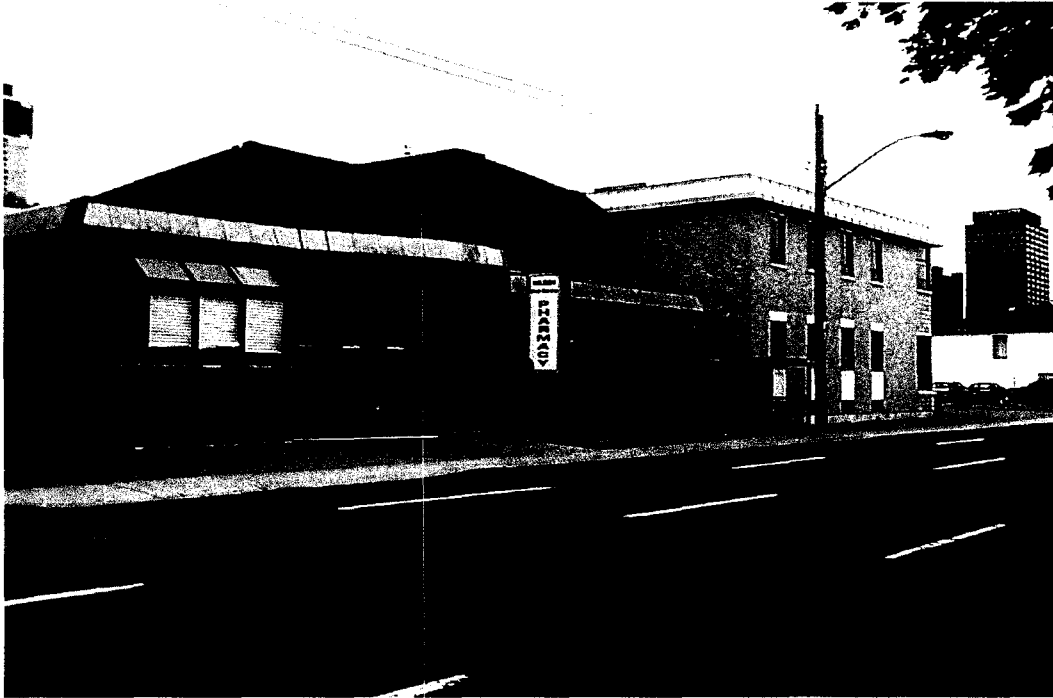
Figure 5.6: Wilson St. Medical Centre
