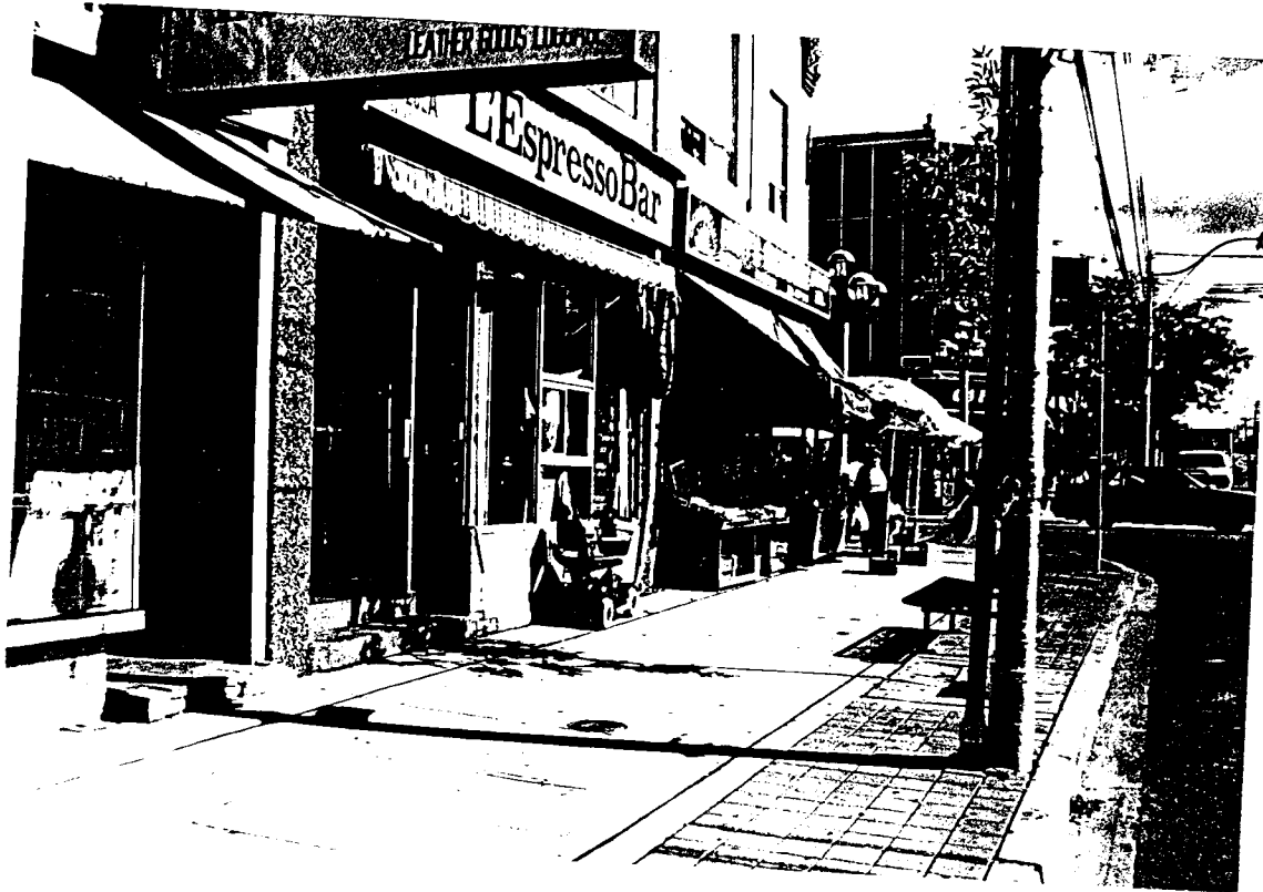
Figure 16: Removal of Vestibule Antonio Ferrantone decided to 'open up' his cafe by removing the formal entrance bay that once centred his property. Now, with the entrance moved to the side, a cafe window is used during summer months to server outdoor patron, while in winter the place-glass is intended to evoke an open air feeling.
