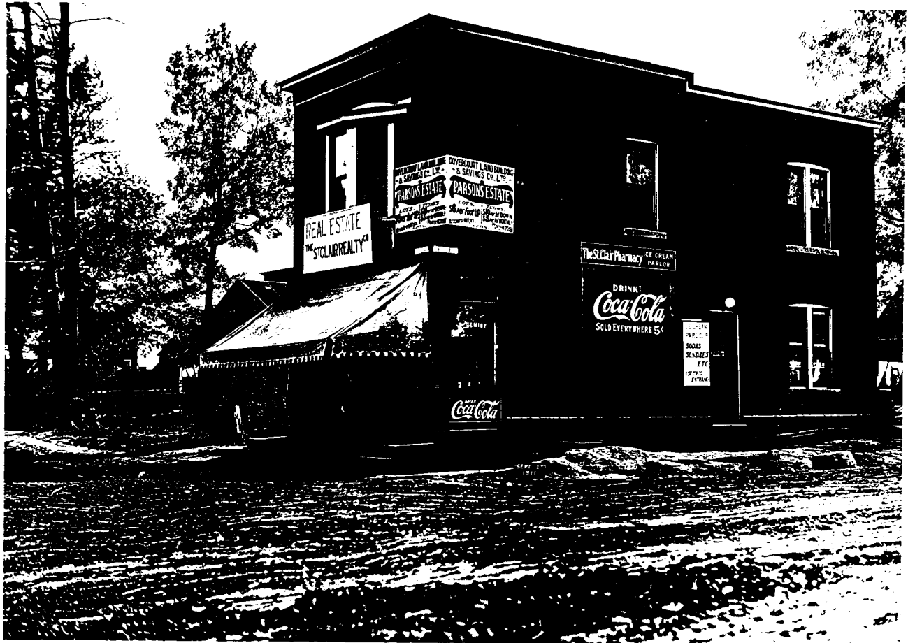
Figure 13: An Original Georgian Structure at St. Clair and Dufferin, 1911. A humble two-part commercial block, many Georgian features are present: dentilled cornice, curved window-heads, stone sills, sliding sash windows, and vestibule. Built before the boom in construction along St. Clair, the building stands alone.
