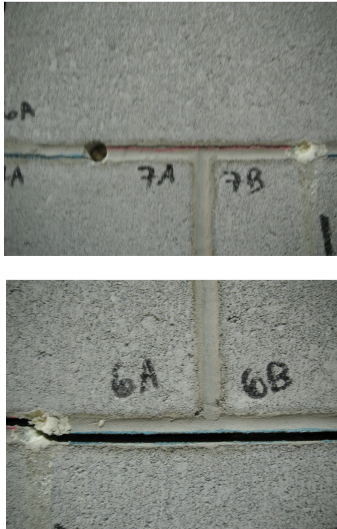
Figure B-0-24: Sudden Widening of Main Crack in High Density C-3 3m Wall
