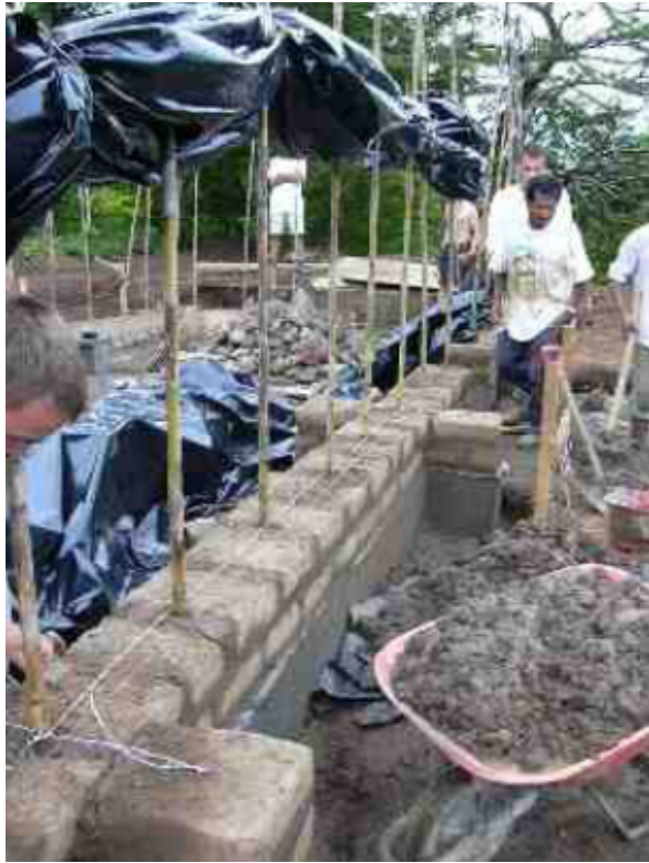
Figure 2-6: Adobe Wall Under Construction with Bamboo Reinforcement (Redman and Smith, 2009)
