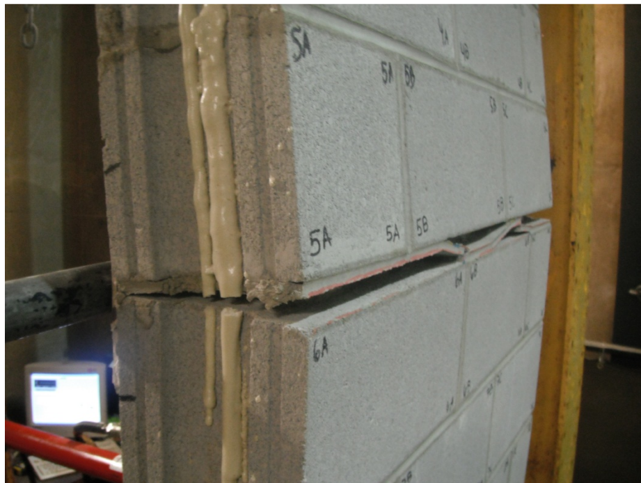
Figure B-0-20: Cracking Pattern of Medium Density C-2 3m Wall
