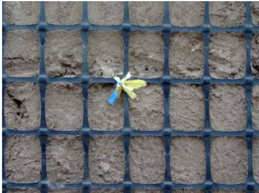
Figure 2-2: Geomesh that is tied to adobe wall (Blondet et al., 2010)
