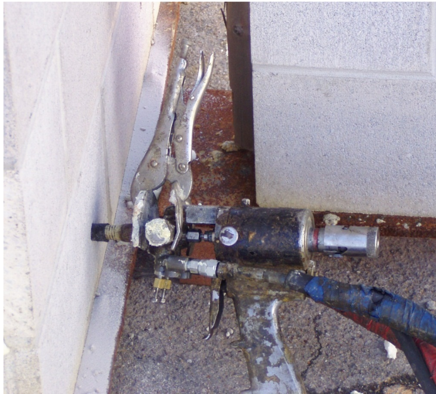
Figure 5-5: Injection Apparatus and Set-up
