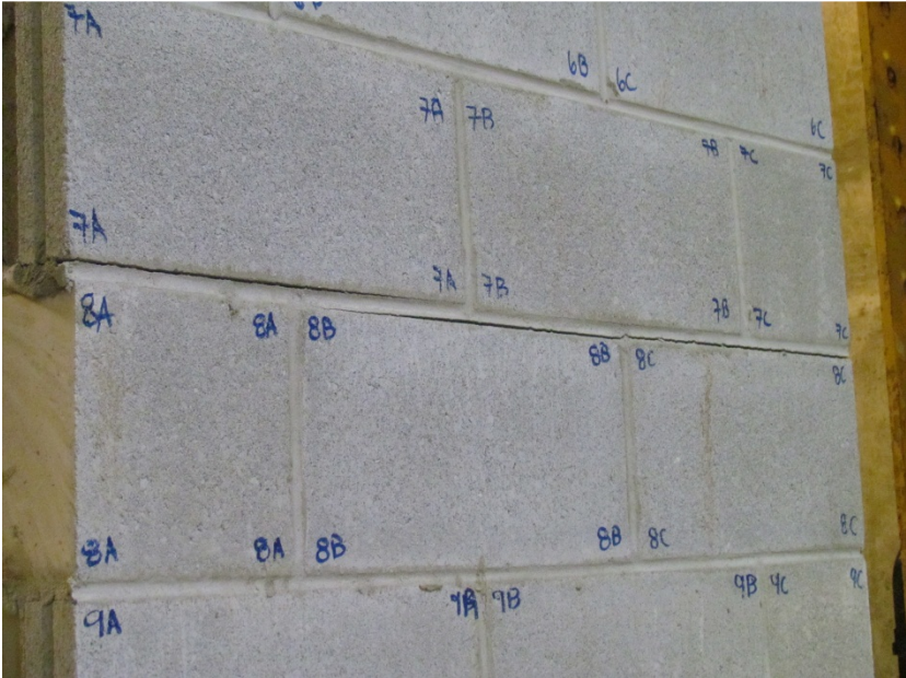
Figure B-0-10: Cracking Pattern of Unreinforced 3 m Control Wall
