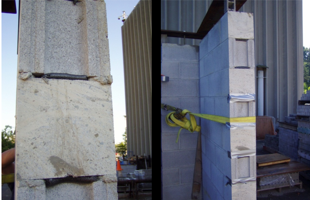
Figure 5-7: Injection Preparation For Walls With Company B Polyurethane Foam
