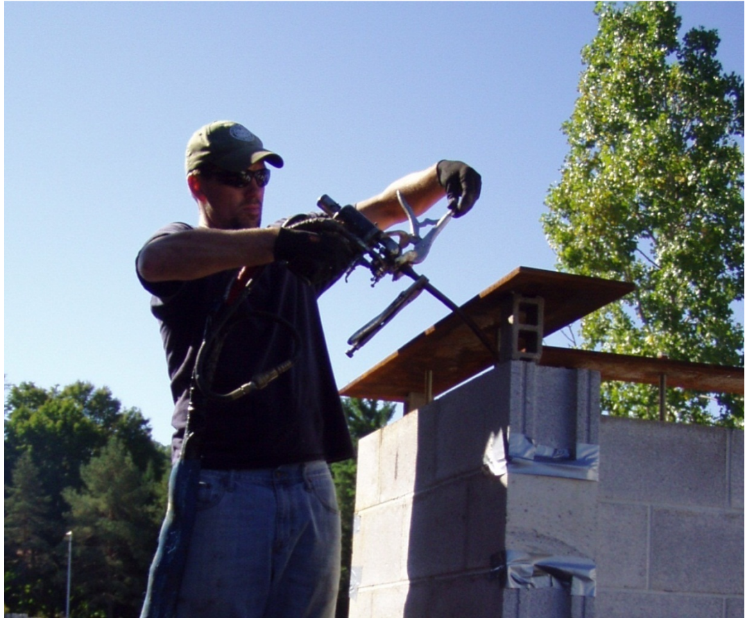
Figure 5-4: Top-Down Injection
