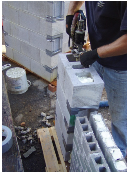
Figure 4-2: Polyurethane Foam Injection into Compression Assemblage
