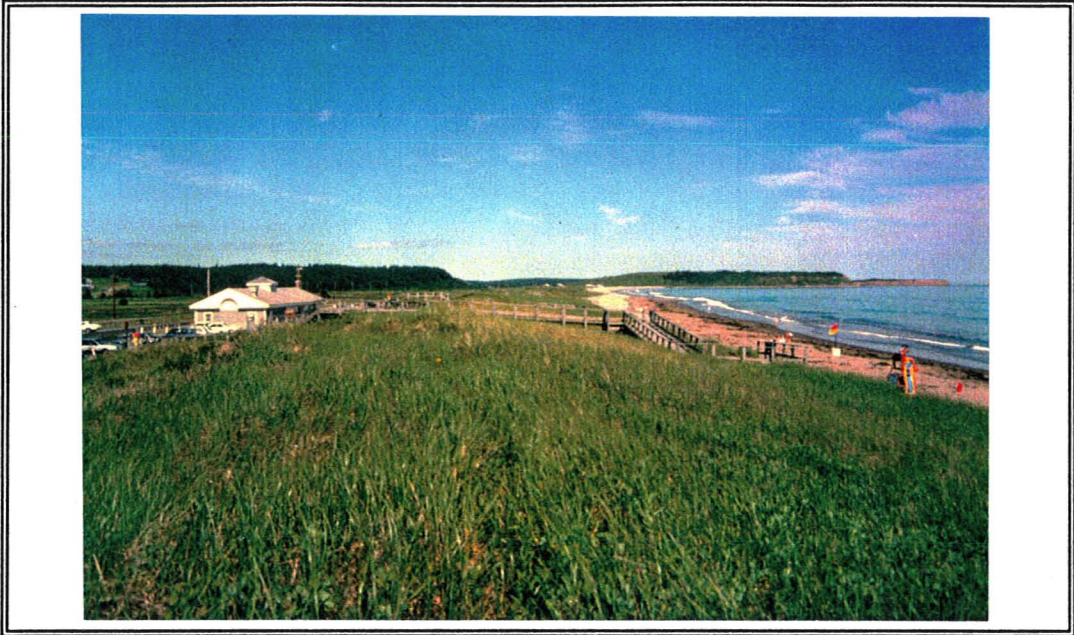
Figure 4.12. Lawrencetown Provincial Park. Note eroding drumlin in distance.
