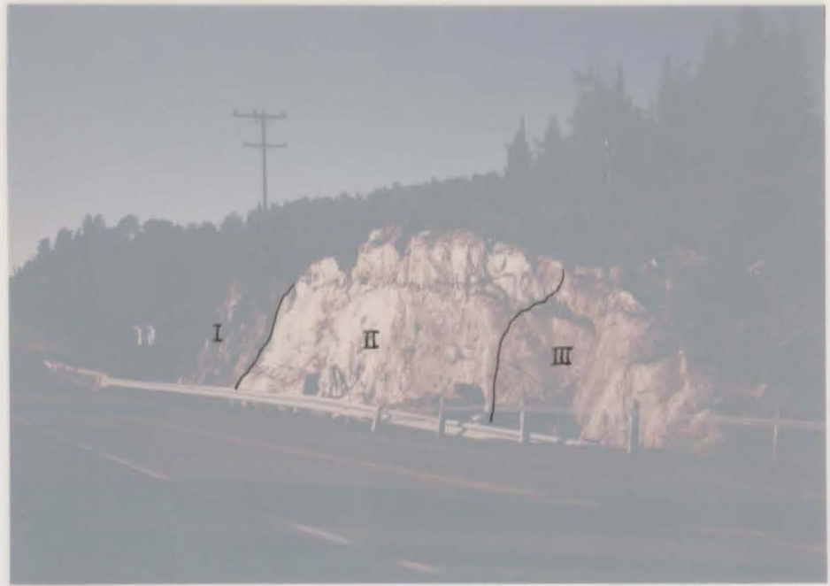
Plate 2. The Misema River Road cut, north face. Sun is reflecting off of foliation planes in section II.
